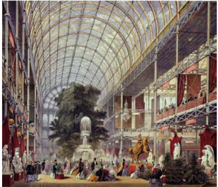
The Crystal Palace (Joseph Paxton, 1851) was made possible by the mass-production of identical elements. The exhibition itself celebrates the mass-consumption of culture.
